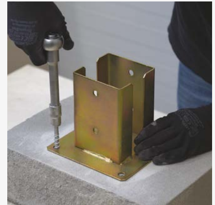
3 Fixing the support into concrete.
