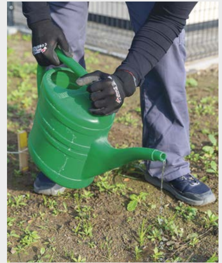
3 Fill the hole with water to allow better feed when screwing in the support.
