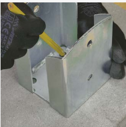
1 Determining hole locations.
