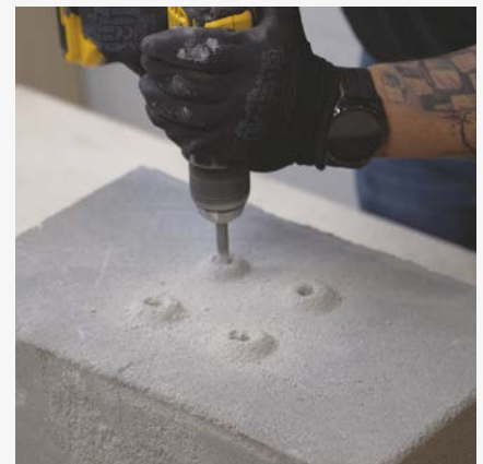
6 Reaming holes in concrete.
