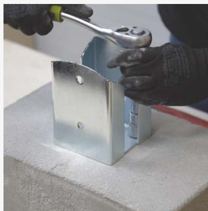
5 Fixing the support into concrete.
