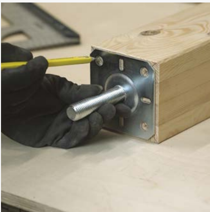
1 Marking the locations for wood screws.
