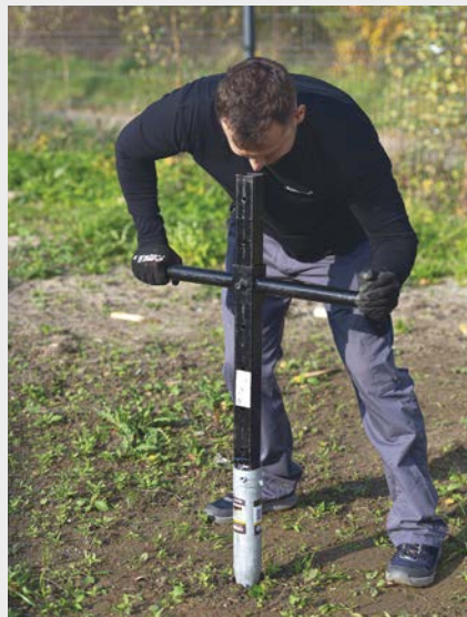
5 Using a metal bar, PWKT spanner or PWPP planetary gear screwdriver, screw the support into the base.
