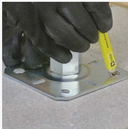
5 Applying the lower support plate and marking out the drilling points in the concrete.
