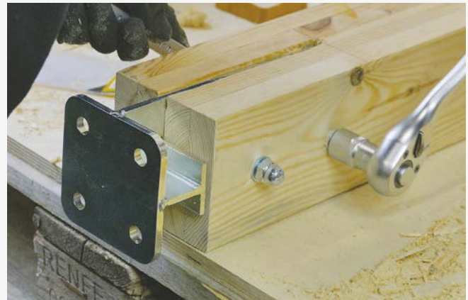
5 Screwing the whole assembly together with nuts using a threaded rod.
