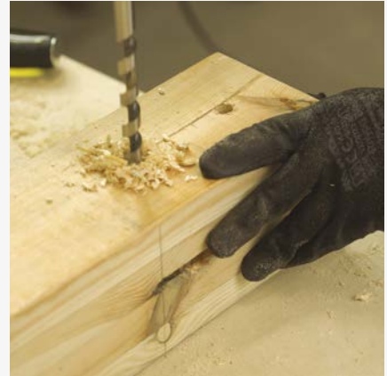
3 Drilling holes through.
