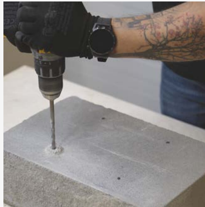
2 Reaming holes in concrete.
