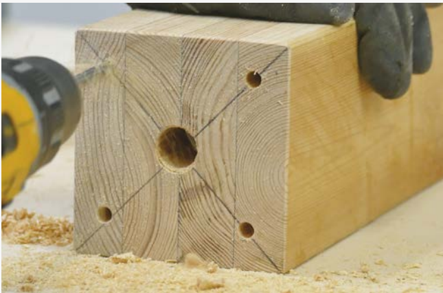
4 Reaming holes for wood screws.
