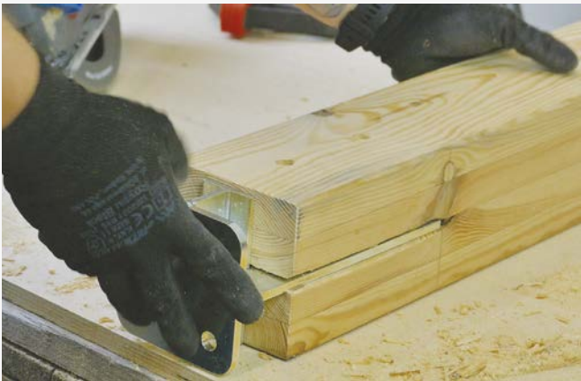
4 Recessing the support into the centre of the post.
