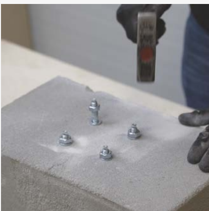
4 Driving in ring anchors.
