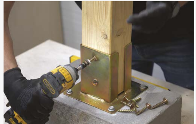
5 Screwing it into the garden structures.
