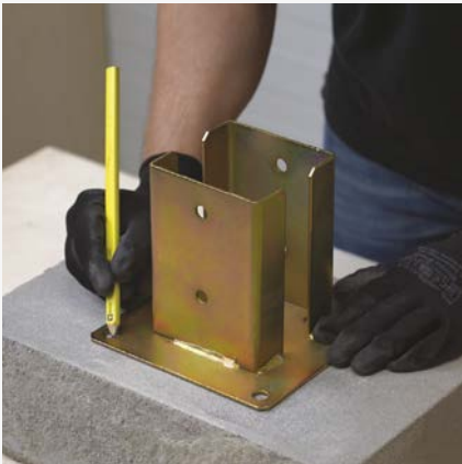
1 Determining hole locations for ring anchors.
