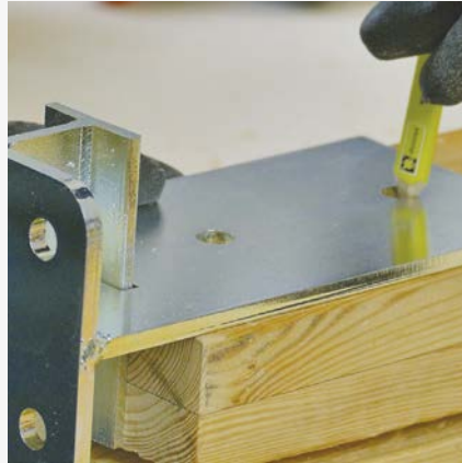
2 Marking out holes for mounting kit for post supports.
