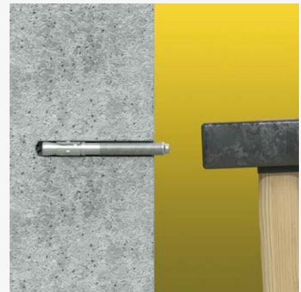
3 Place the anchor in the drilled hole.
