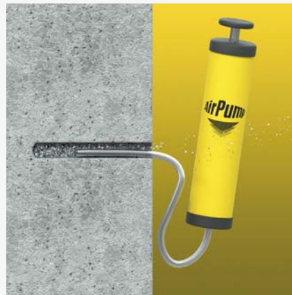
2 Clean the hole of dust and dirt (using a pump or a brush).
